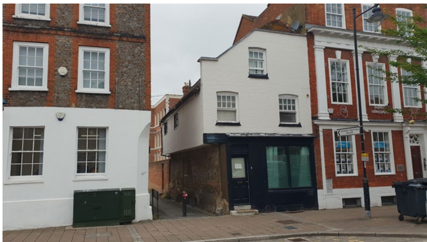
Figure 13: Medieval Back (15 th ) / Georgian (18 th ) shopfront, London Street, Reading. (Source: RBC Planning).
