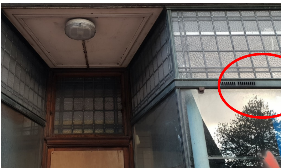
Figure 34: Photo of historic façades, with air grilles in Friar Street. (Source: RBC Planning).
