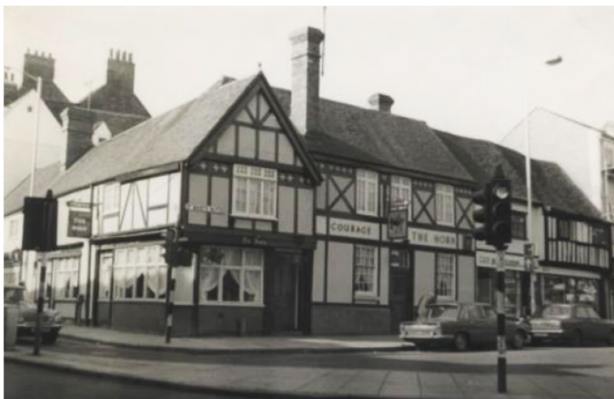
Figure 41: 1979 The Horn. Public House. St Mary's Butts, Reading. Source: RBC Planning
