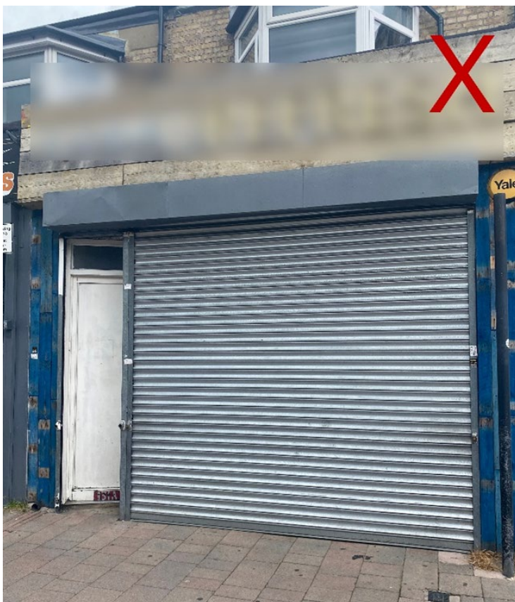
Figure 48: Shopfront with solid external security shutters (not in Reading) (Source: RBC Planning).
