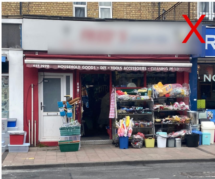
Figure 42: Shopfront with cluttered forecourt (Source: RBC Planning).
