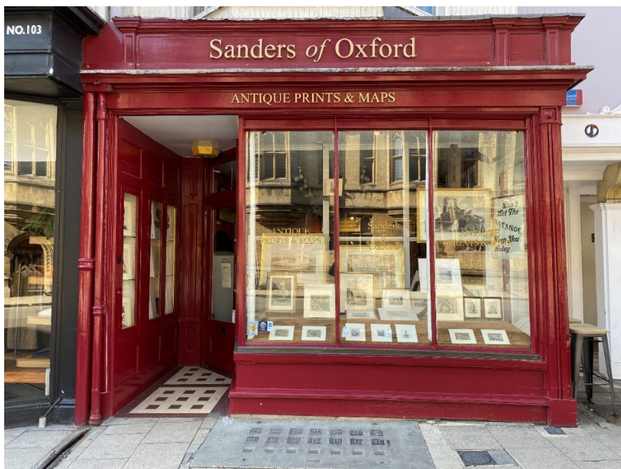
Figure 52: Shopfront with traditional recessed entryway at High Street, Oxford. (Source: RBC Planning).
