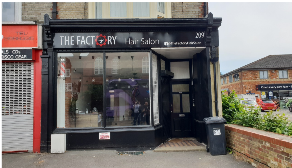
Figure 38: Good example of signage, on Oxford Road, Road. Note a well detailed timber glazed black shopfront. Source: RBC Planning
