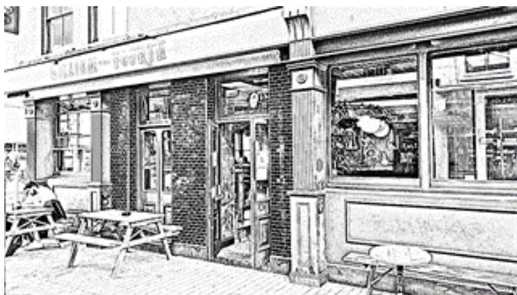
Figure 53: Panelled, plain and fluted pilasters with decorative consoles. Brighton. (Source: RBC Planning).
