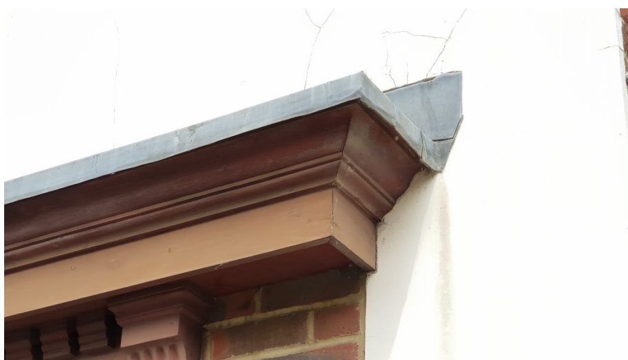
Figure 50: Cornice with lead flashing over, Reading. (Source: RBC Planning).
